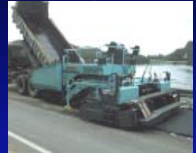
Asphalt pavement material, etc
