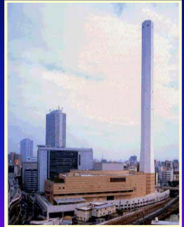
Toshima incineration plant (capacity:400t/d) (power generation capacity :7,800kW)
